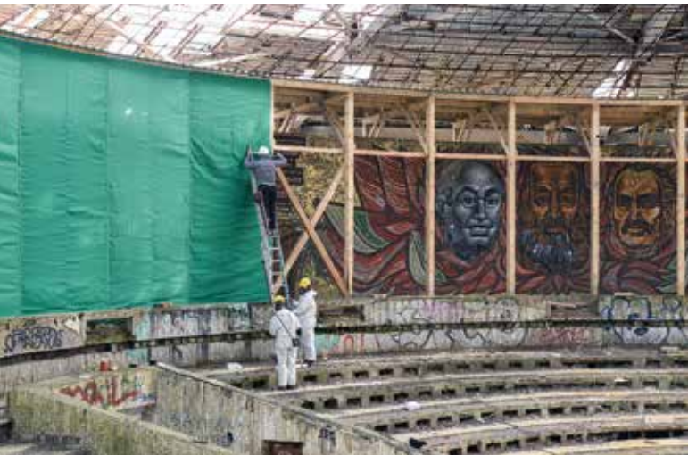
Fig. 2 Main Hall, inner ring during the enclosure works, 2020
