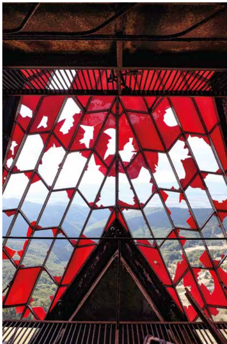
Fig. 1 The twelve-metre five-pointed star from the pylon at Buzludzha, made of glass and metal, current state
