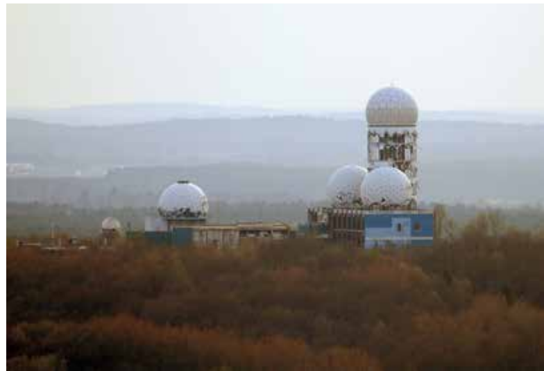
Fig. 5 Berlin, former wiretapping installations on Teufelsberg, photo A. Savin, 2013
