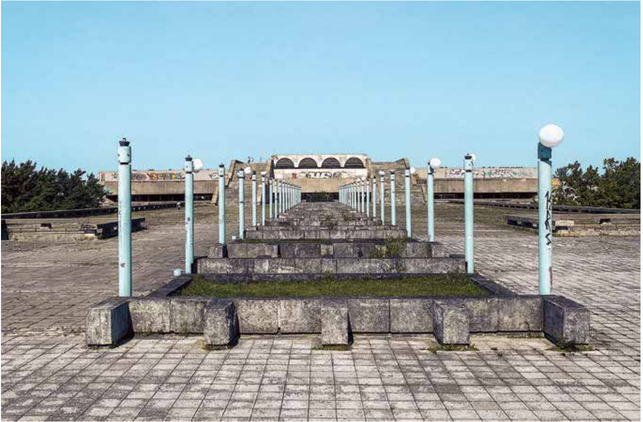
Fig. 3 Linnahall, photo from the Visit Tallinn marketing album “Tenet Location in Tallinn”
