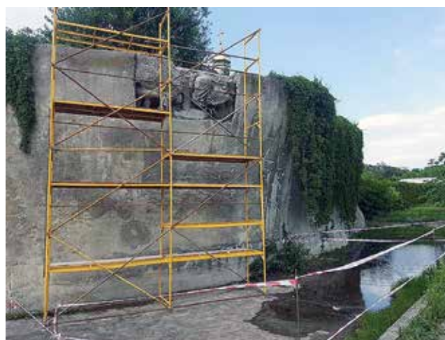
Fig. 1 A part of the concrete top layer was removed in 2018, revealing the relief of a face gazing upwards
