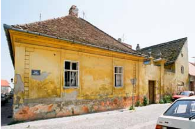
Fig. 13-11: Osijek, Miller's house, state before renovation 1996
