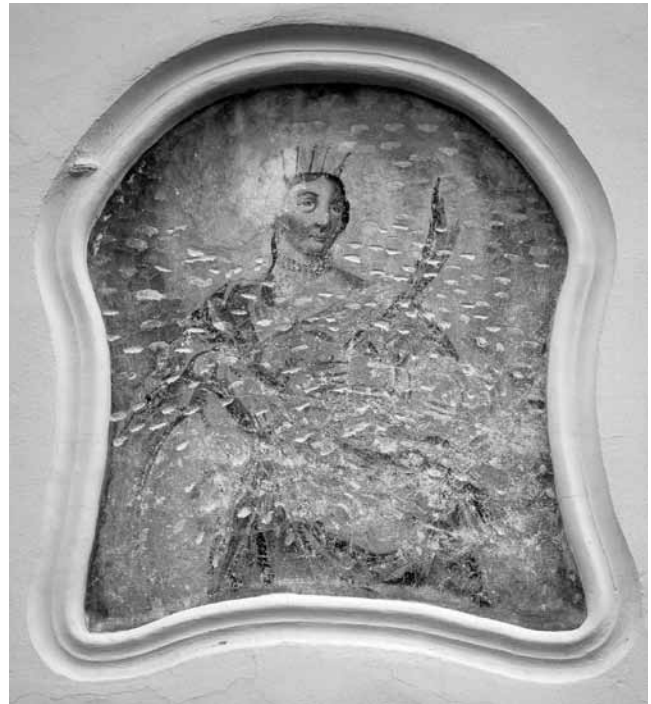
Fig. 13-3: Varaždin, Fresco painted on western façade of the house in Gajeva st. 16 (Paraloid B72), state in 2011
