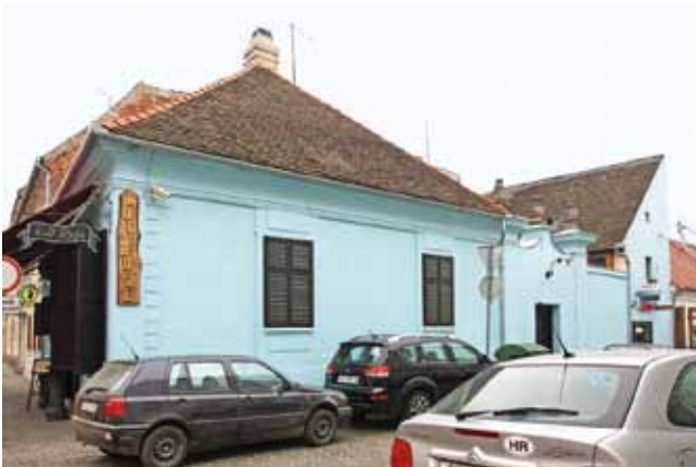
Fig. 13-12: Osijek, Miller's house with the old plaster and paint layers below the new paint, state in 2011
