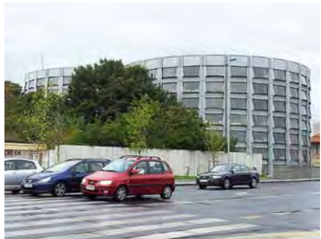
Fig. 11: The Garage in Ljubljana showcases the architect's innovativeness in building technology and structure, which was constantly researched in the projects of Savin Sever, 1969
