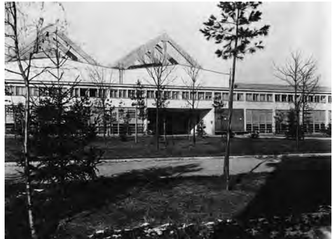
Fig. 3: The Litoštroj factory was a large-scale industrial plant, designed as an open structure in green surroundings, with innovative building structures to present the enforcement of the new society in industrial development. The metalworking plant has a suspended roof fixed on triangular brackets. Architect: Miroslav Gregorič, 1946
