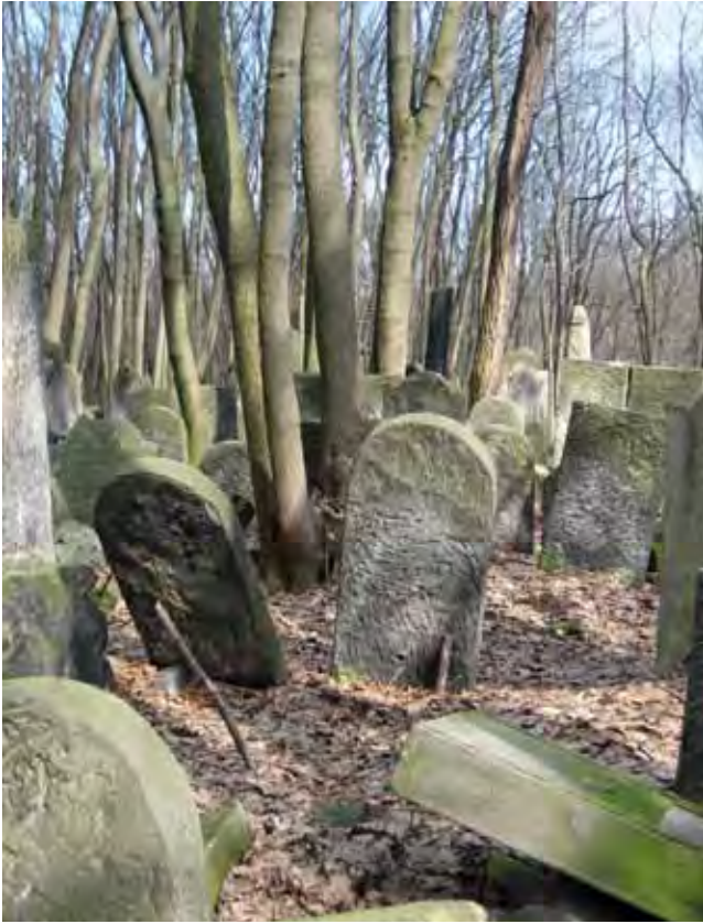
Fig. 4 Falling tombstones demonstrating tree-derived neglect of the burial ground, Okopowa Street Cemetery, 2011 (photo by E. Nekanda-Trepka)
