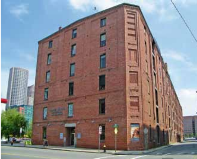
Figure 11: Patterned brick at the corner does little to relieve the plainness of the Atlas Stores, FPCD, the first part of which was built in 1890 by BWCo
