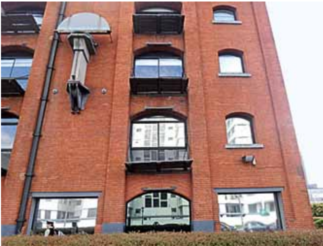
Figure 9: Detail of restored façade
