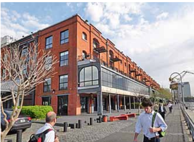
Figure 8: Pedestrian promenade along the dock
