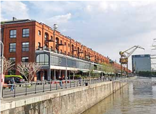
Figure 7: Warehouses on the western bank
