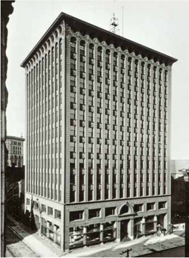
Figure 4: Exterior, Guaranty Building (1894–96), Buffalo, N. Y., Adler & Sullivan
