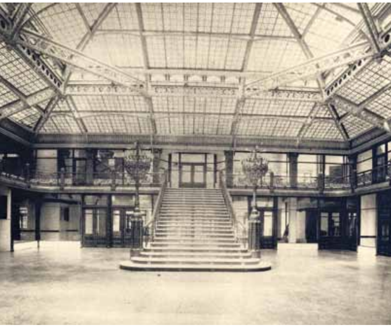
Figure 8: Interior, The Rookery (1885–1888), Chicago, Burnham & Root
