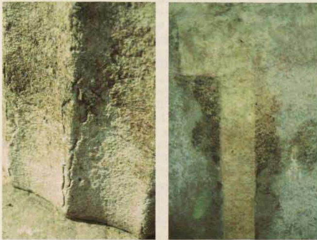
Fig. 14a-b. Milet, marble columns: Surficial carbonate precipitation mainly caused by the metabolic activity of photosynthetic algae and cyanobacteria (a) and different cleaning treatments (laser, mechanical and chemical procedures) to remove the aesthetical detrimental crusts (b).
