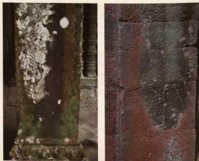
Fig. 12a-b. Angkor, temple complex, details: Natural multicoloured biofilms of different photosynthetic microorganisms (i.e. lichens, algae and cyanobacteria), distinctly separated due to expositional factors and interspecific competition.
