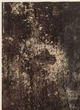
Fig. 2. Zadar, Cathedral of St Anastasia (Sv. Stošija), south apse, wall painting, detail: typical deterioration of paint layer.
