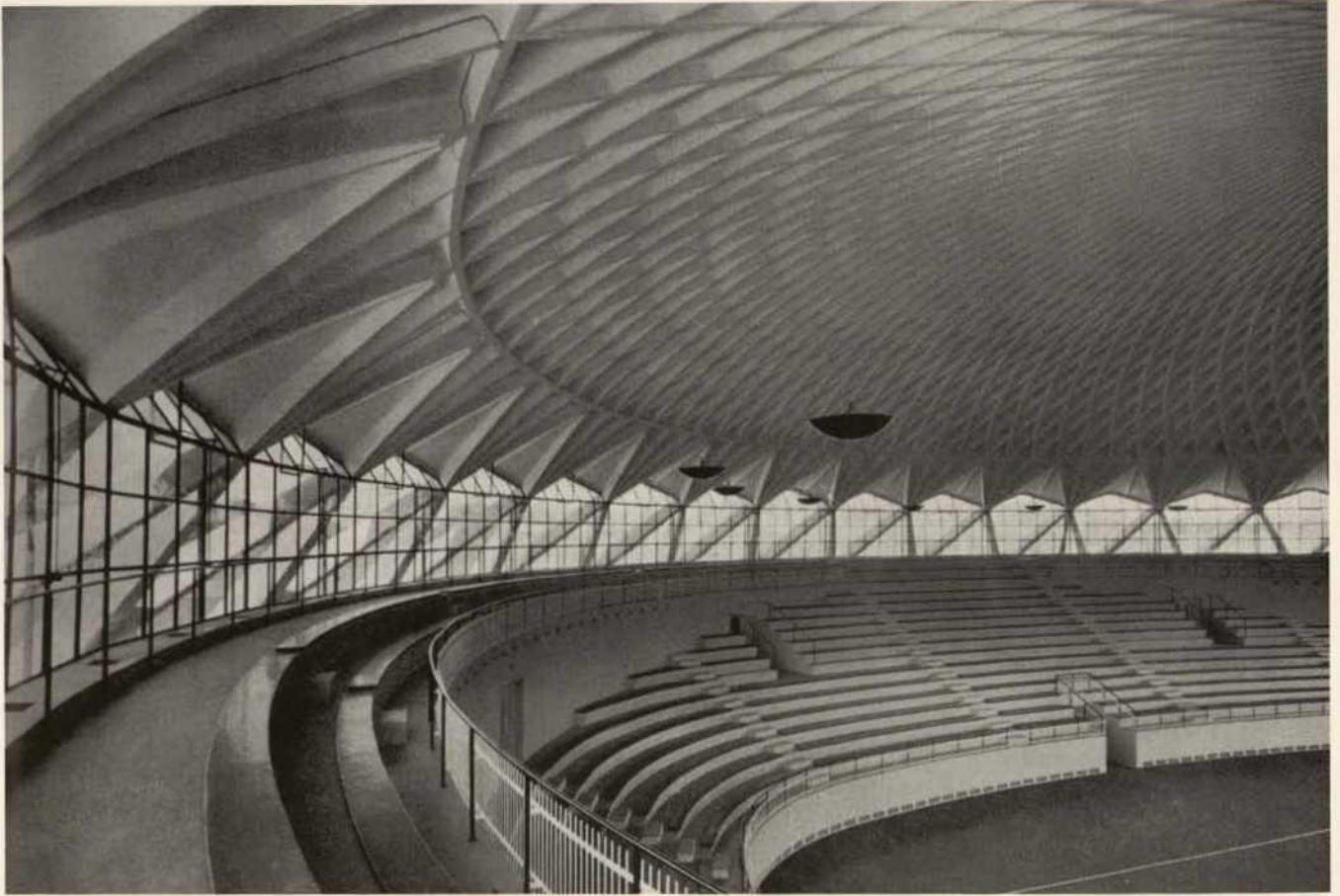
Fig. 11: Pier Luigi Nervi and Annibale Vitellozzi, Palazzetto dello Sport in Rome (1956-58). Detail of the seat rows and of the „cupola“ which covers the hall. The „cupola“ is composed of 1620 pre-cast reinforced concrete sections with 19 different sets of dimensions.
