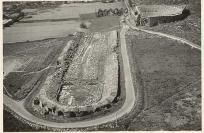
The well preserved Stadium of Perge (Pamphylia Region)
