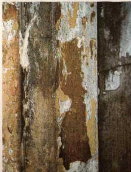
4 Fragment of a stone window frame, the first window from the south. Multi-layer polychromy clearly visible with delaminating yellow layer of 19th-century over-painting; state before restoration in 1998 (Photo by S. Musiela)
