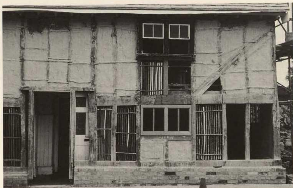
Fig. 2. Repairs using Traditional Materials. – The owner of this cottage wanted to use traditional materials to repair it. New materials can sometimes have a role in repairs, but the advantage of traditional ones is that they have been tested over hundreds of years.
