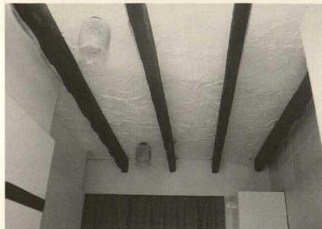
Fig. 7. Fake Beams at Highpoint. – The Society strongly opposes fakes. Here fibreglass beams have been stuck to the ceiling of one of the most important examples of a 1930s building in Britain. However they are removable.
