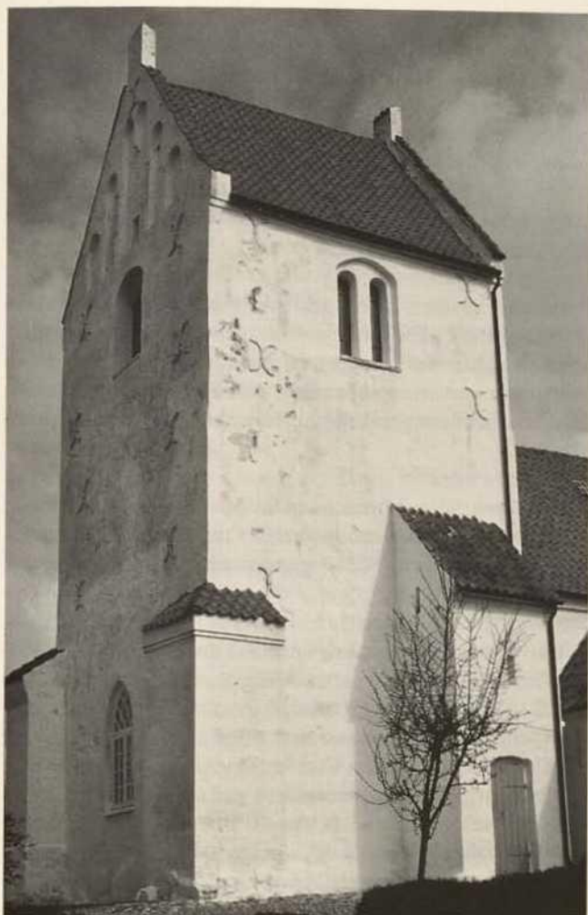
Fig. 7. Vallekilde Church (Zealand) 1996. The rendering has fallen off in the areas with cement and hard-burnt bricks. Repairs have later been executed with hydraulic mortar, which seems to hold.
