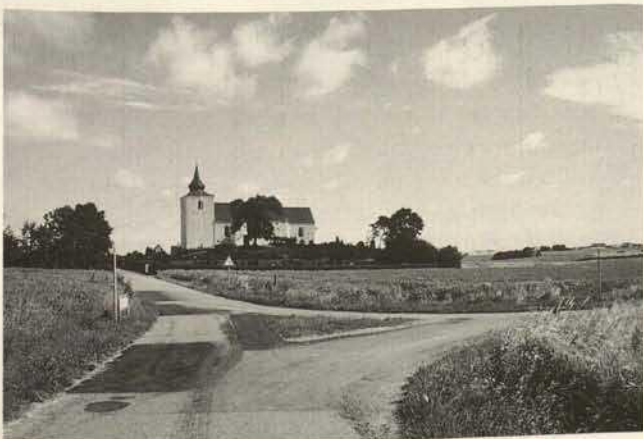
Fig. 1. Ølsted Church (Jutland). Romanesque apsis, chancel and nave built of calcareous tufa. Tower and porch are late medieval and made of bricks. Limewashed.
