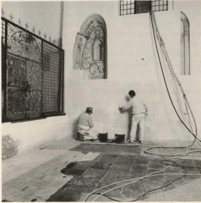
Fig. 10. Århus Dome. Masons limewashing undecorated areas under guidance of a conservator.
