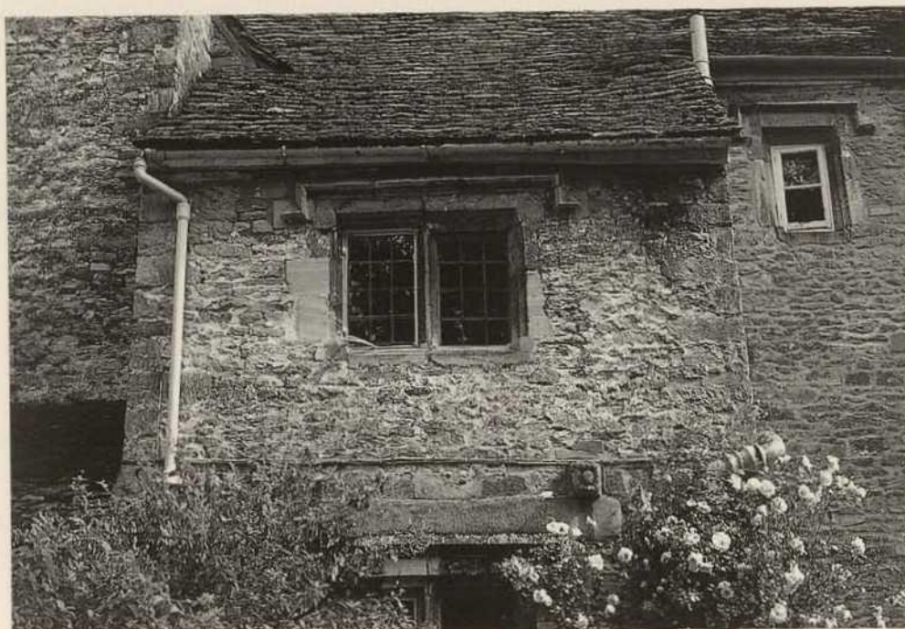
Fig. 6. Second case study: Woolgatherers staircase. The original lime surface before repair work. Note previous repairs with Portland cement on wall to right, and on timber lintel below.
