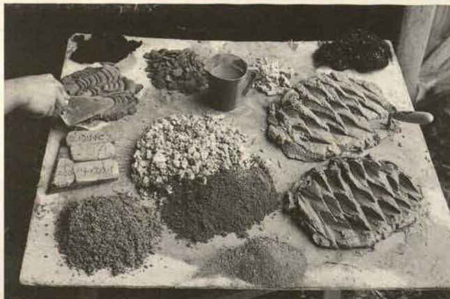
Fig. 9. Third case study: Broadfield Court. The range of lime products used on the repairs to the doorway. Note goat hair for reinforcement of mortar for hoodmould.
