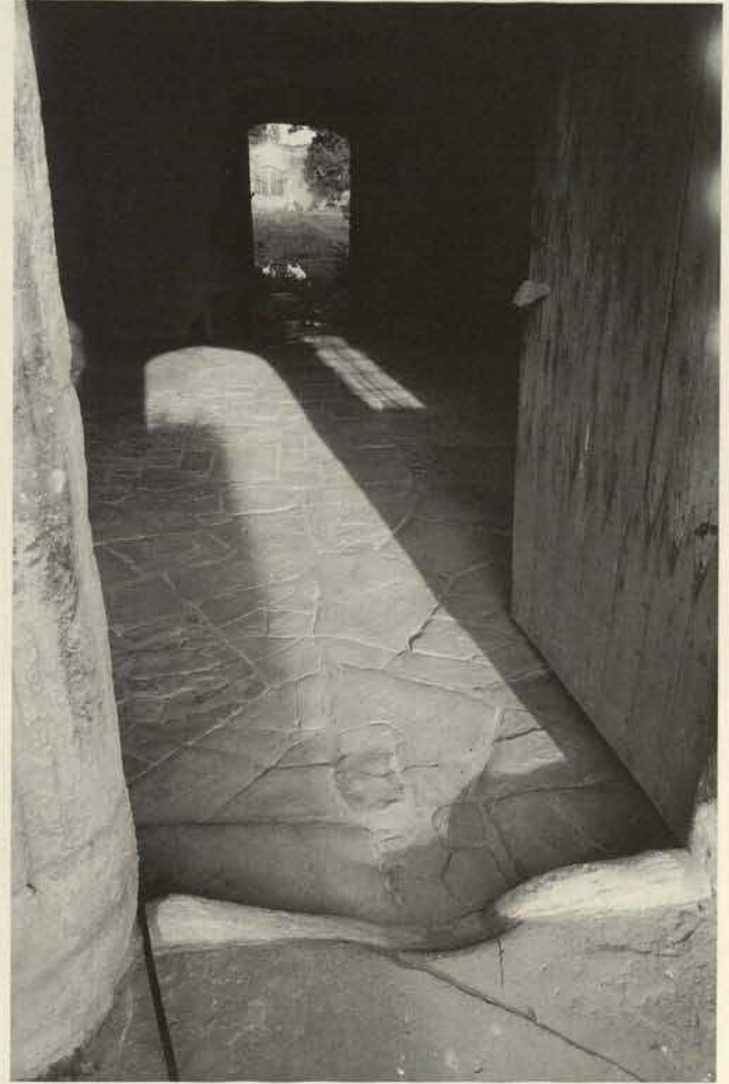
Fig. 12. Fourth case study: Acton Court. Cross passage floor from west to east after lime mortar repairs. Note the unusual configuration of pennant stone parving.
