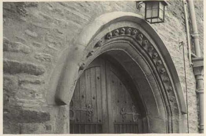
Fig. 10. Third case study: Broadfield Court. The completed lime repairs. Note the limewashed stones of the hoodmould, and repointed rubblework.
