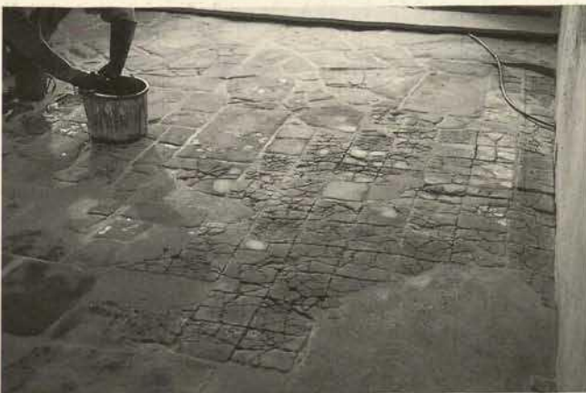
Fig. 11. Fourth case study: Acton Court. Cross passage floor after lime repairs. Note lacunae filled with mortar, and only the larger joints.
