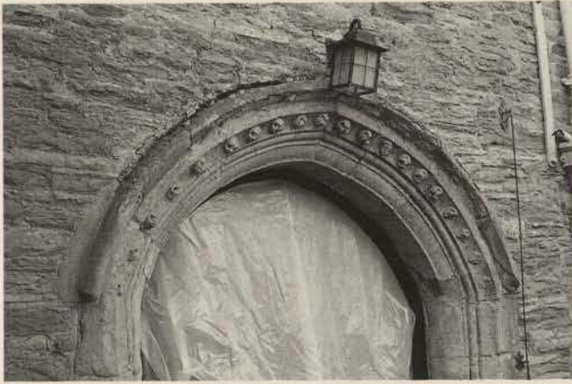
Fig. 8. Third case study: Broadfield Court. The fourteenth century doorway before repairs. Note decayed surfaces to hoodmould and surrounding rubblework, and Portland cement fillings.
