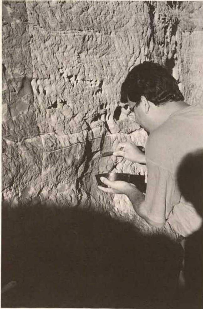
Fig. 4. Mortar application in test field C
