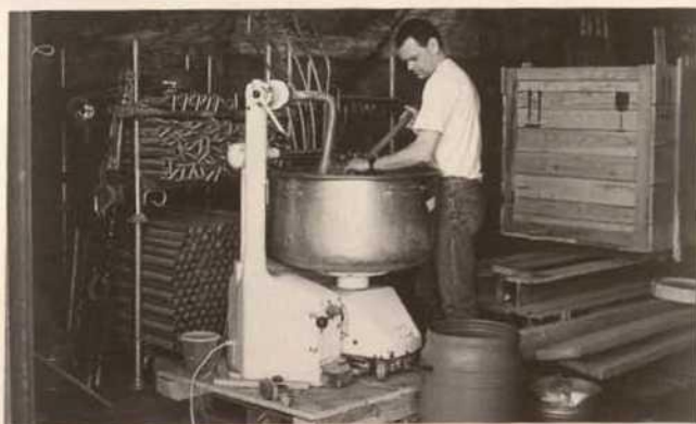
Fig. 6. Restorer Egon Kaiser preparing repair mortar on the heaving-arm-kneader (mixer)
