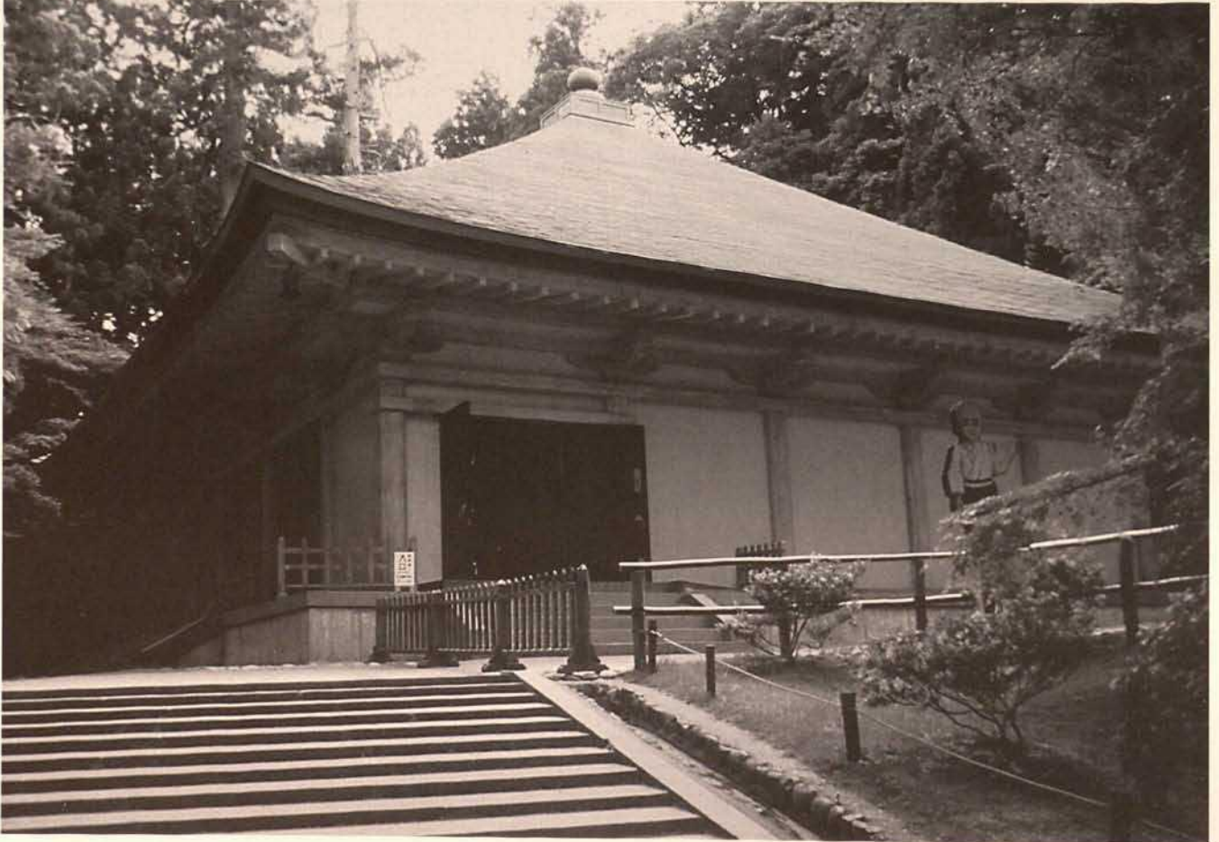
Fig. 1. View of the present shelter
