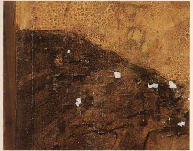
2 Damage of the historical gloss lacquer on the marbled altarpieces of the Church of the Holy Cross at Landsberg. The details show the extent of yellowing and alligating caused by the recent lacquer coating after only six years, additions also caused the here visible delaminating and losses of polychromy
