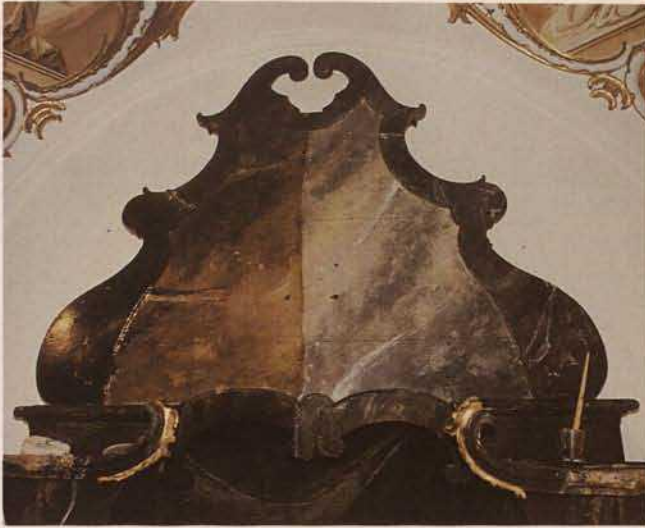
1 Top of a marbled side altarpiece in the Convent Church at Roggenburg, with remains of the historical gloss lacquer on the left, which has already been removed on the right half. Condition report during the restoration 1983–1985
