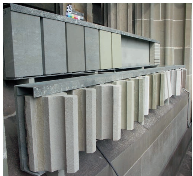
Fig. 2. Test samples with various mortar mixtures, surface treatments and joints were exposed to the weather on all four sides of the tower, at the level of the intermediate gallery.
