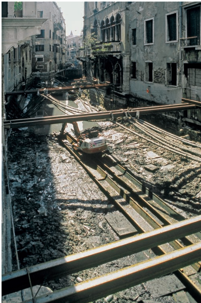
Fig. 5. Cleaning of the canals and rehabilitaiton of substructures.
