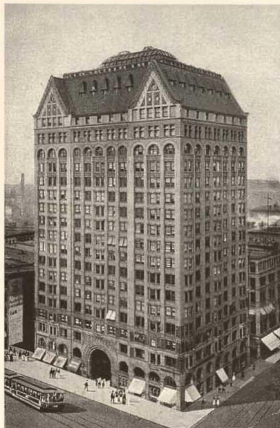
III, 4 Chicago, historic view of the Masonic Temple (Burnham and Root, 1892). This building, now demolished, utilized a steel frame that was laterally stiffened with a diagonal bracing system and did not rely on the masonry curtain wall for lateral support as had earlier skyscrapers.
