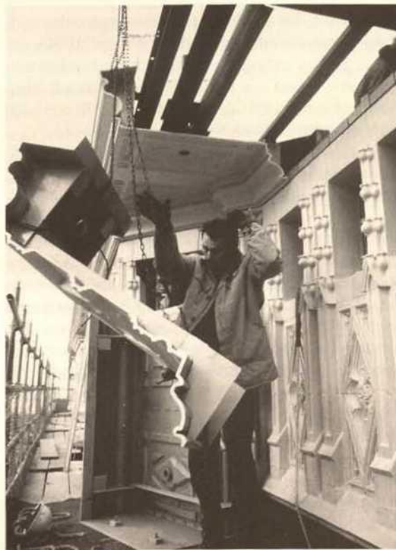
III, 5 Chicago, Reliance Building: During terra cotta replacement exposed metal elements such as columns, spandrel beams, and the cast iron mullion and rail system, were cleaned and painted. It was found that the mullion and rail system was in relatively good condition. If this system was found to be significantly deteriorated the restoration project would not have been feasible. (left)
