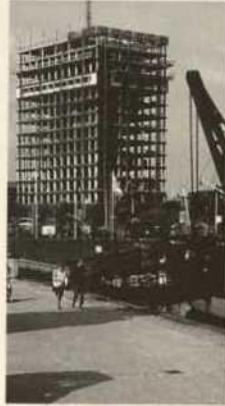
III. 1 Rotterdam, Blaak 333 during its renewal (1987-1992)
