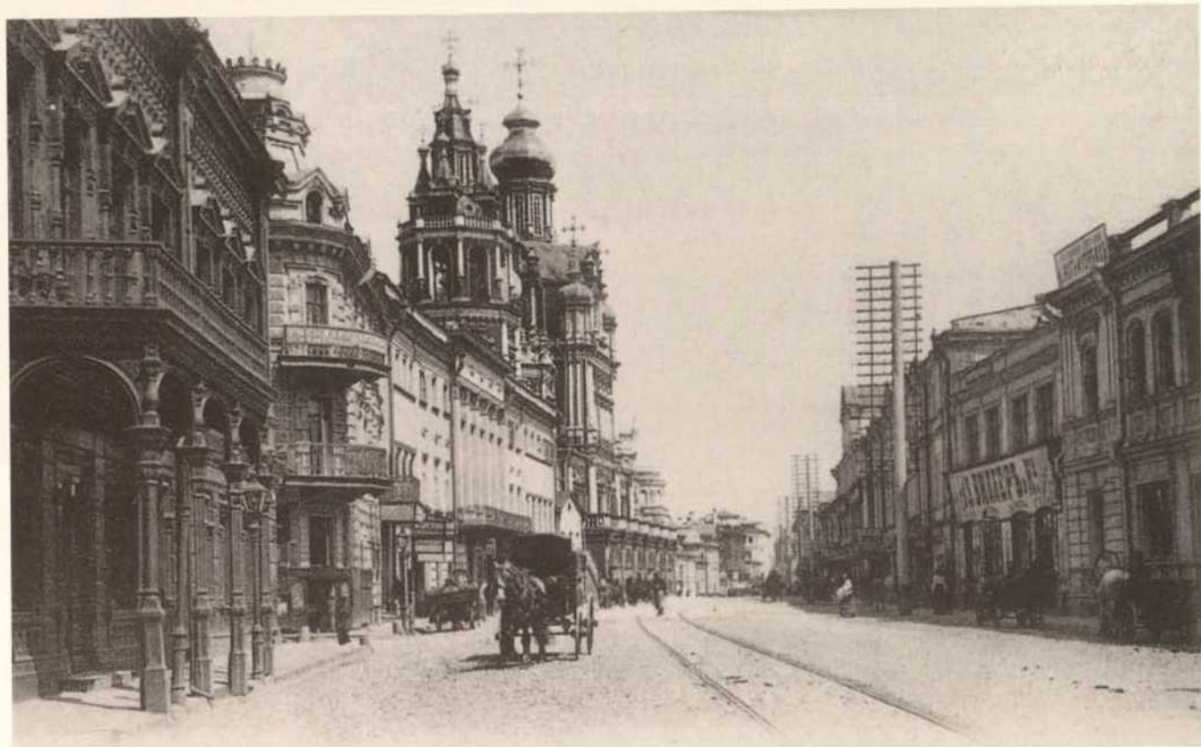
St. Virgin's Assumption in Pokrovka street (Moscow 1696-1699), an outstanding building of the Russian 17th century, destroyed in 1936
