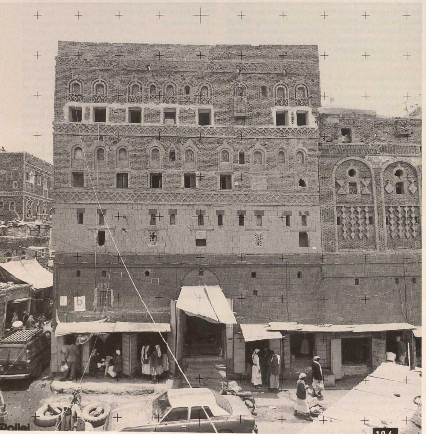
Abb. 2. Samsarat al-Mansurah; Ostfassade, Rolleimetric-Photogrammetrie; 1988 Fig. 2. Samsarat al-Mansurah; east façade; 1988
