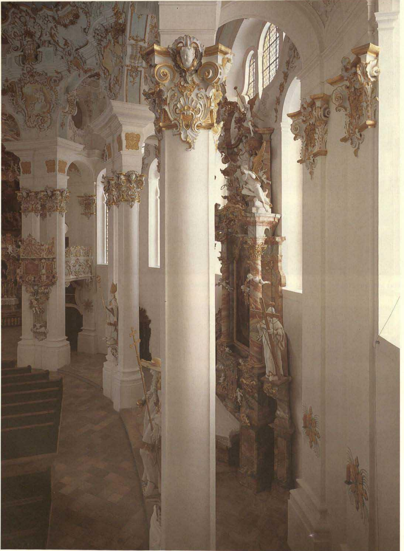
Blick in den südlichen Umgang des Gemeinderaums / View in the south ambulatory of the congregational space
