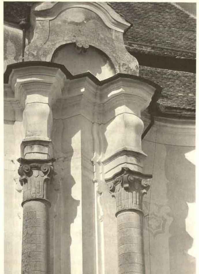
Fig. 12. Exterior facade, pair of columns at the junction with the entablature
