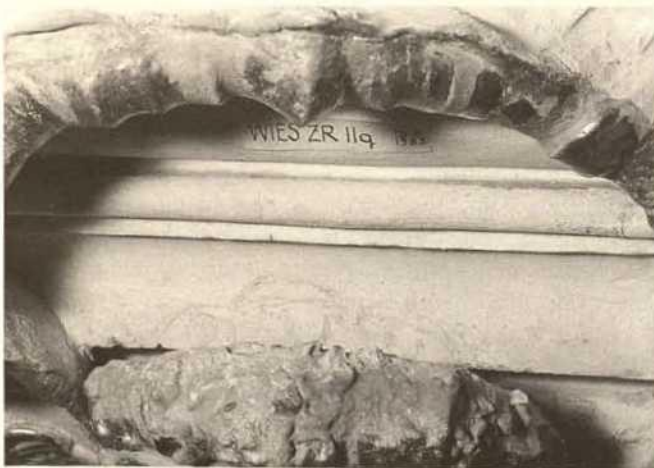
Fig. 15. Cornice on cartouche q; preliminary drawing in pencil for the stucco work
