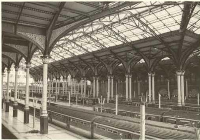
Ill. 1. The interior of the trainshed at Liverpool Street Station, London, designed by E. Wilson, 1874-5, following its refurbishment by Nick Derbyshire.
