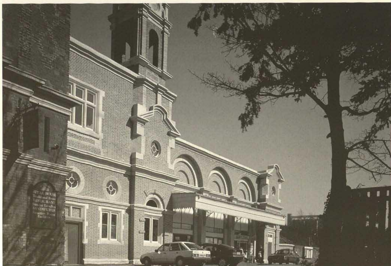
Ill. 9. Bury St Edmunds, Suffolk, was threatened with demolition. Local people fought fiercely to save it and it has now been restored and cleaned with the help of a grant from the RHT.
