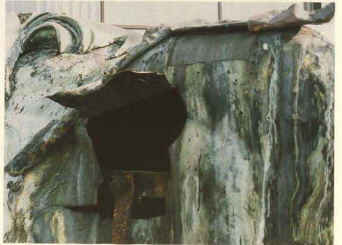
2a, b. Prague, corrosion manifestation on the sculpture Genius with a Lion (A. Popp, 1937)
