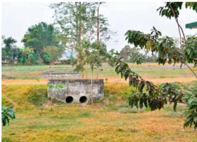
Fig. 5: Road as embankments (2014)
