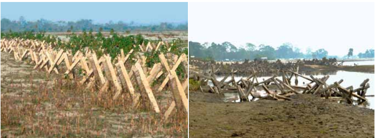
Fig. 7: R.C.C. Porcupines before & after the floods of 2013
