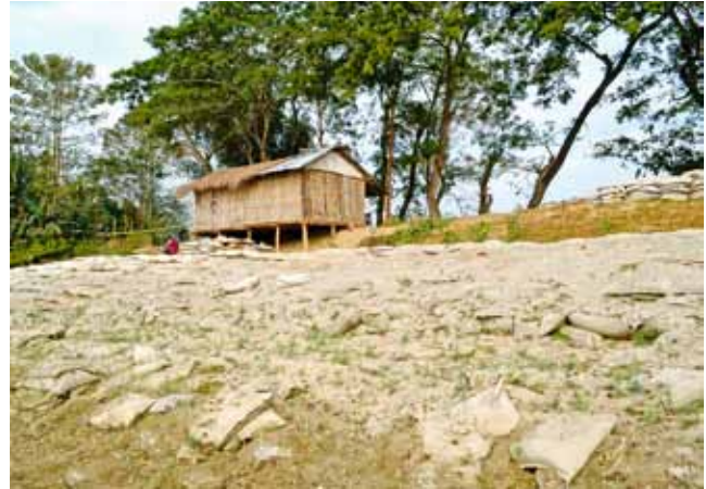
Fig. 4: Ineffective measure, river bank after the floods (2014)
