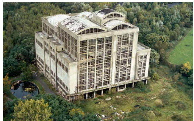
Fig. 9: Péronnes-lez-Binche – the sorting and washing rig
