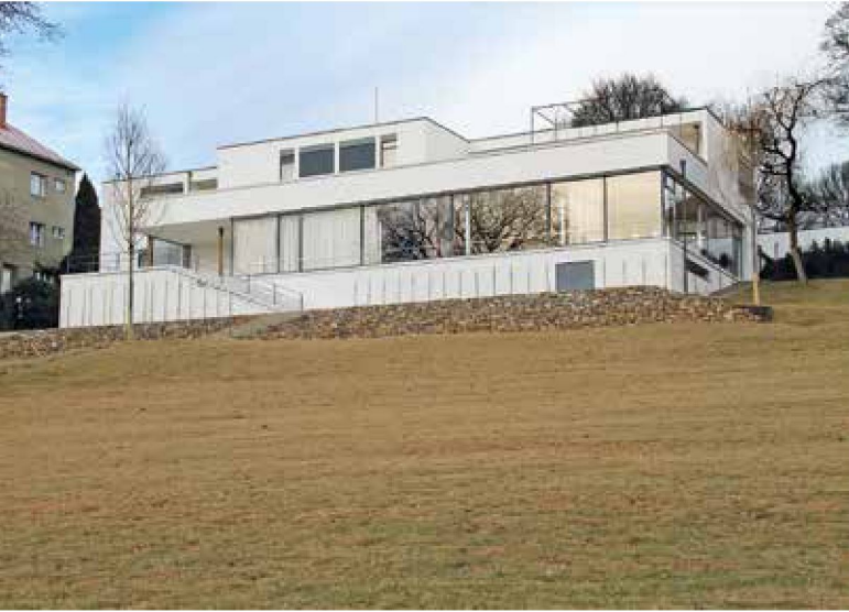
Fig. 2: The Tugendhat House after restoration work, 2011
