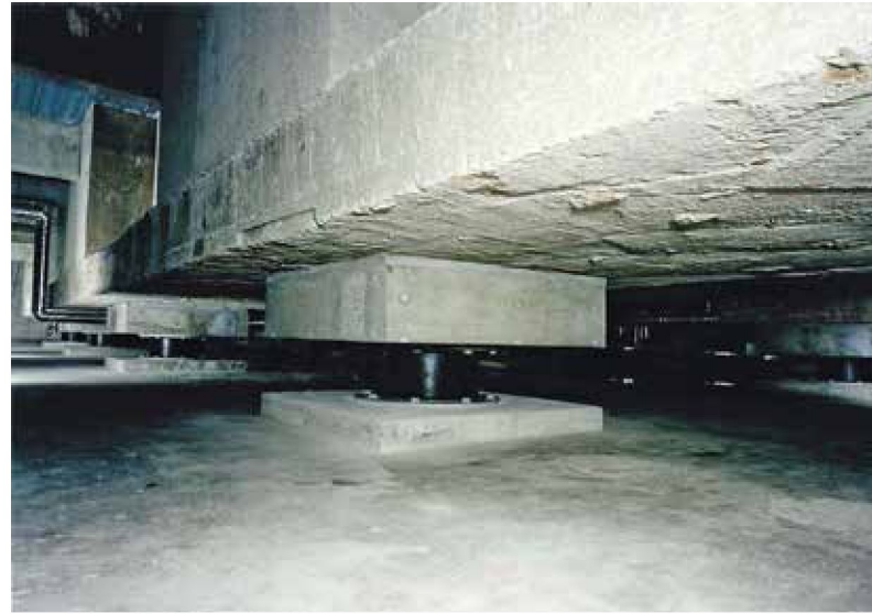
Fig. 13: National Museum of Western Art, Le Corbusier, 1959; seismic isolation retrofit
