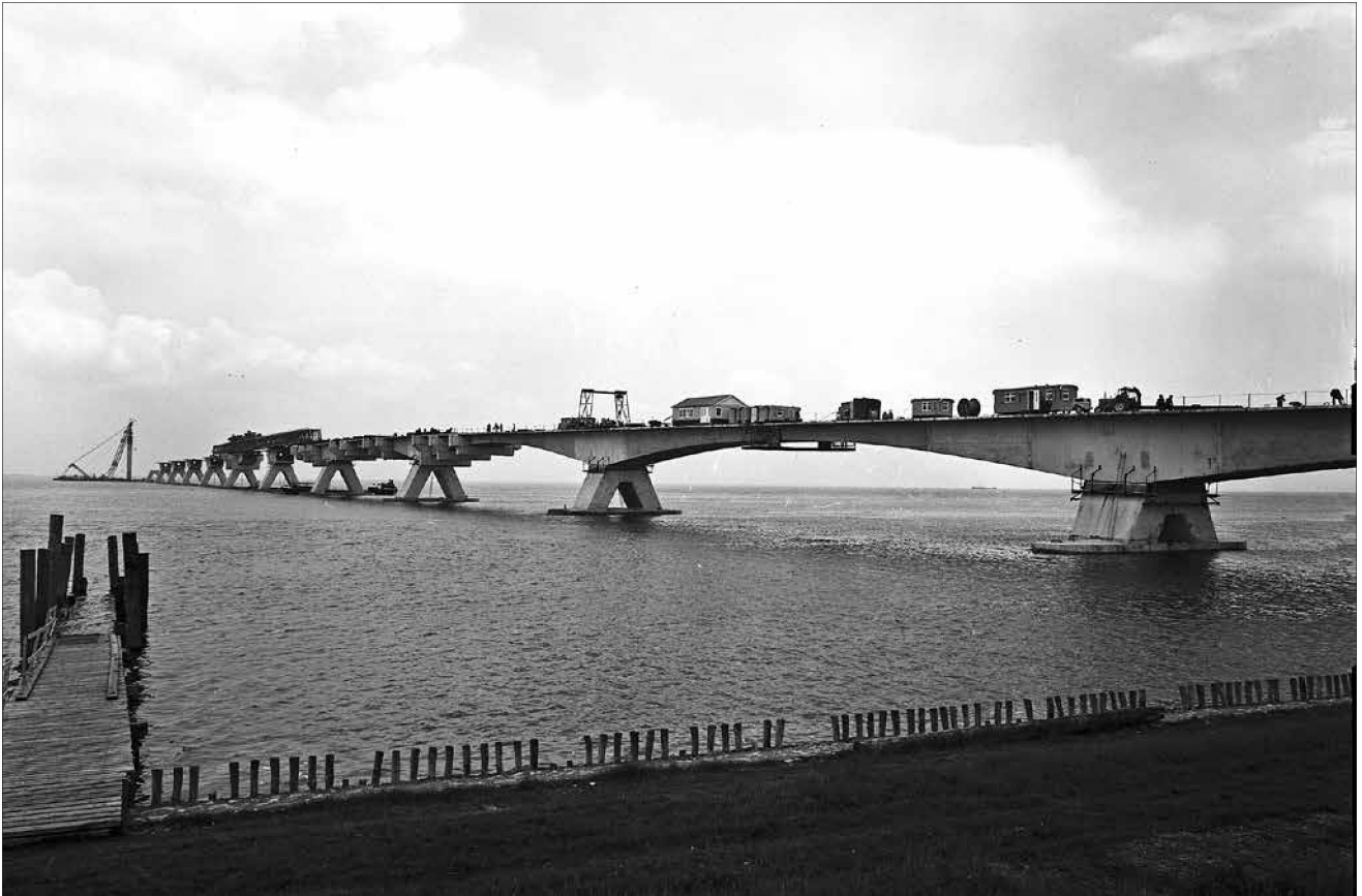
Fig. 8: Zeeland Bridge under construction
