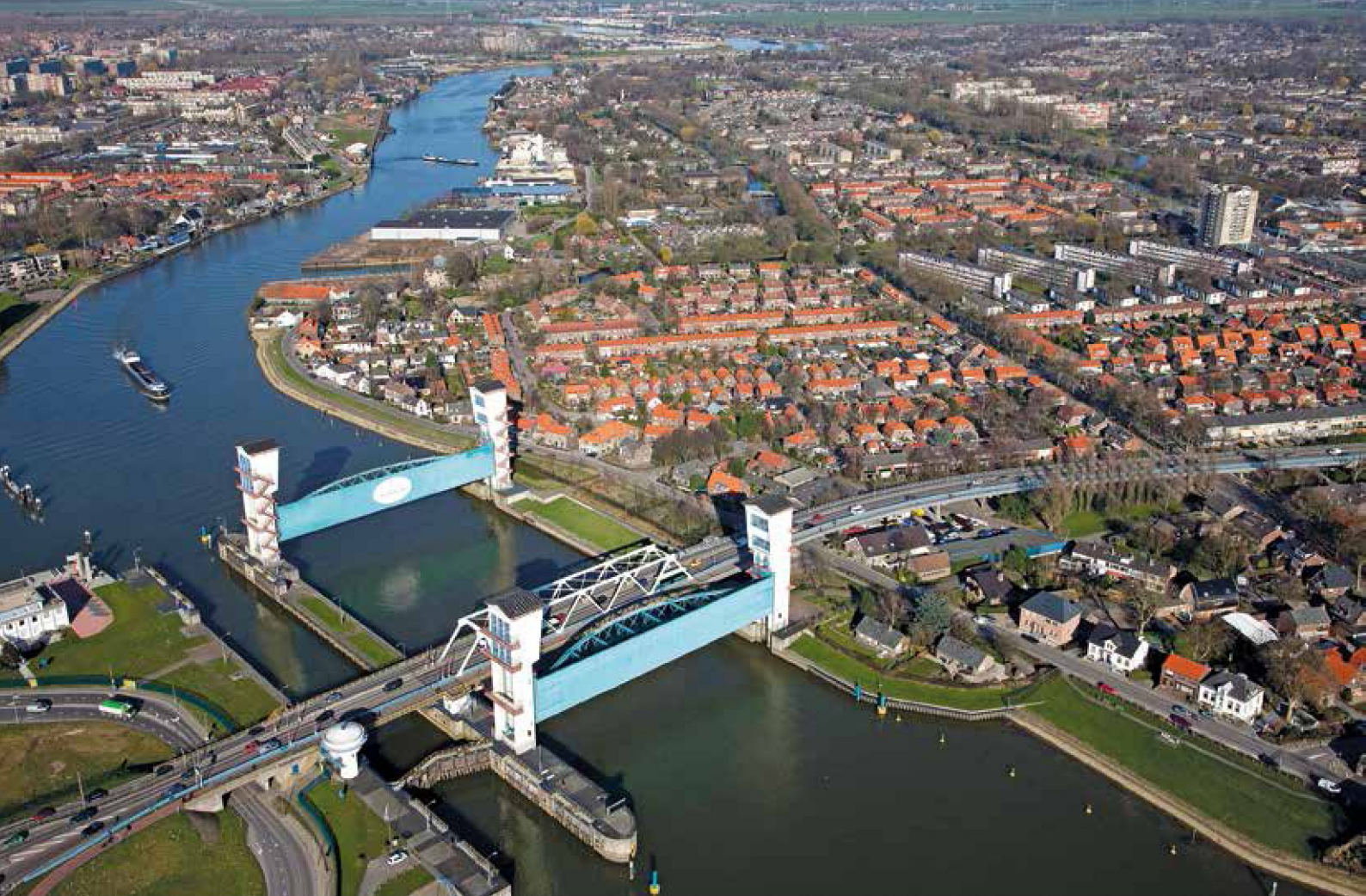
Fig. 4: Storm Surge Barrier Hollandse IJssel from the air
