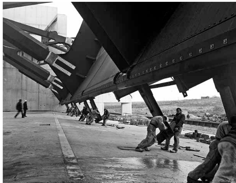
Fig. 6: Haringvliet discharge sluices under construction
