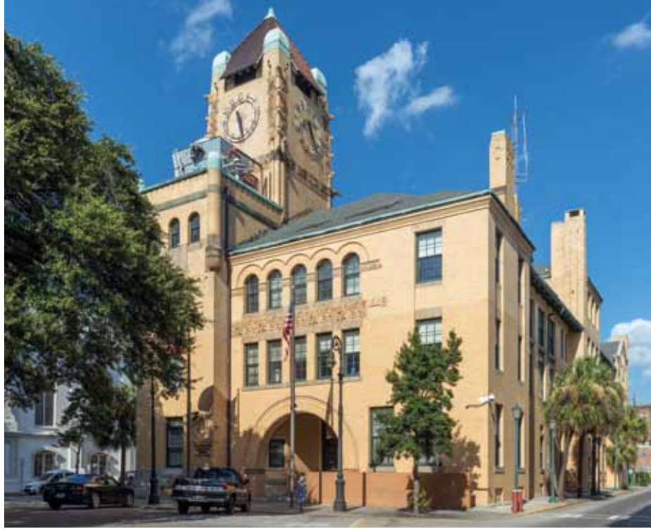
4 William Preston, Chatham Courthouse, Clocktower, Savannah, Georgia, 1889 (status 2016)
