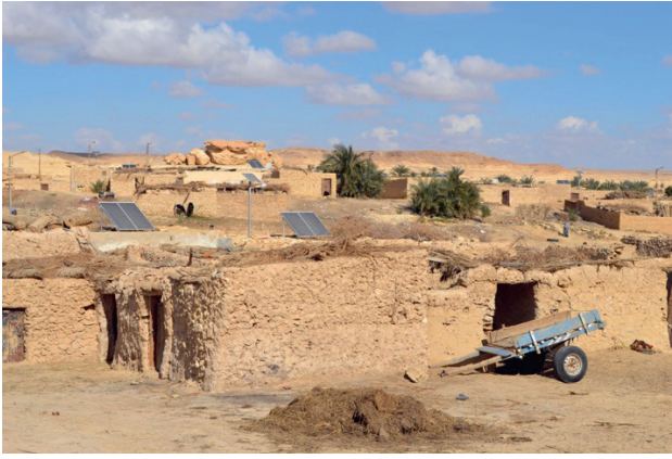
Fig. 5 Al Gara village in Siwa after retrofitting one of its vernacular buildings with PV systems for electricity production (photo: Nahla Makhoulf)
