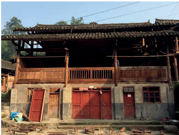
Fig. 7 (b) Wooden roof trusses and eaves without fire-resistant coating in entire Dali Village
