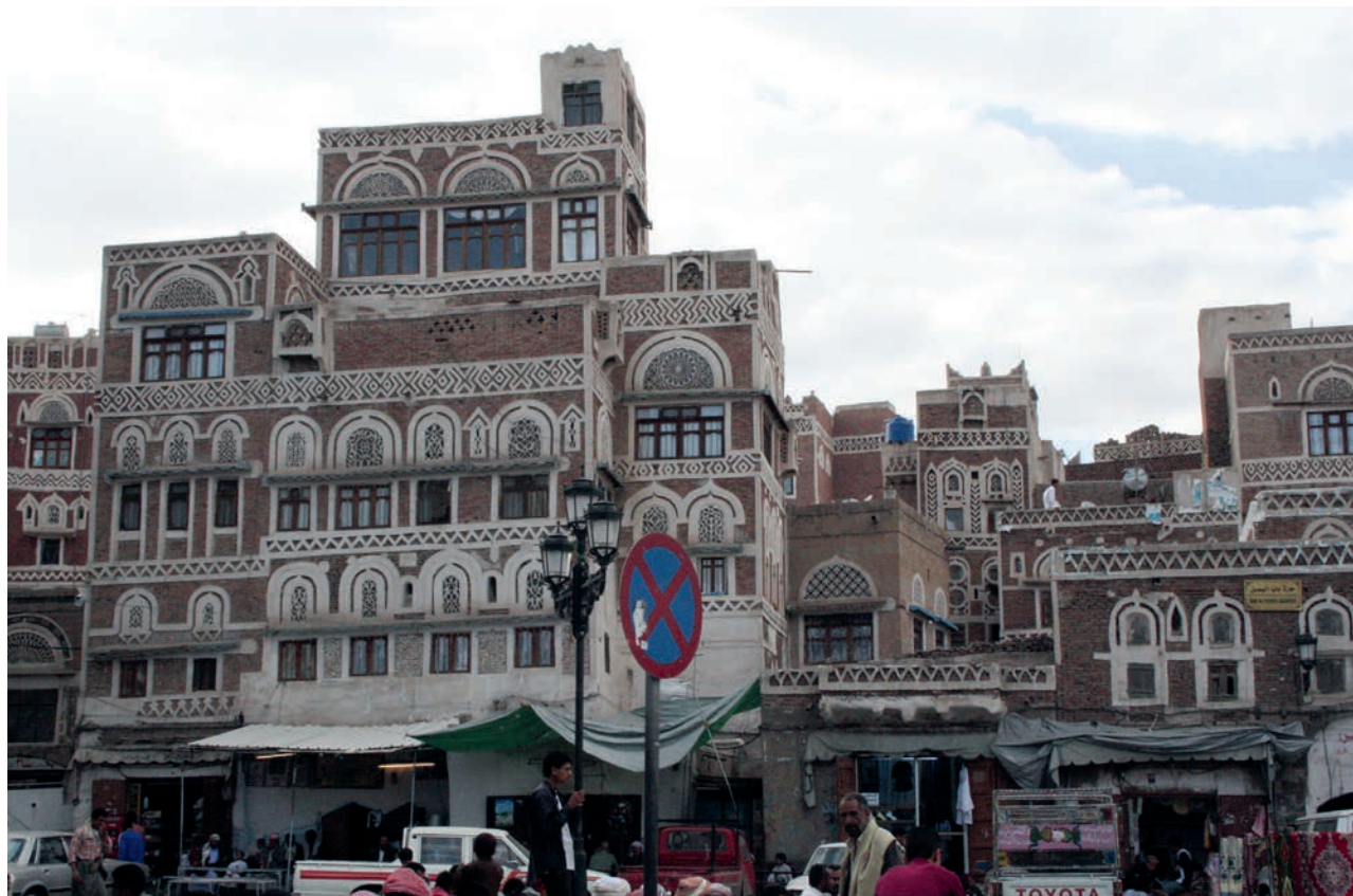
Fig. 1 Traditional houses in 'Suq al-Malh', Sana'a, Yemen (the Old City of Sana'a was inscribed on the World Heritage List in 1986), a wealth of vernacular built heritage threatened by war (© Hossam Mahdy 2007)
