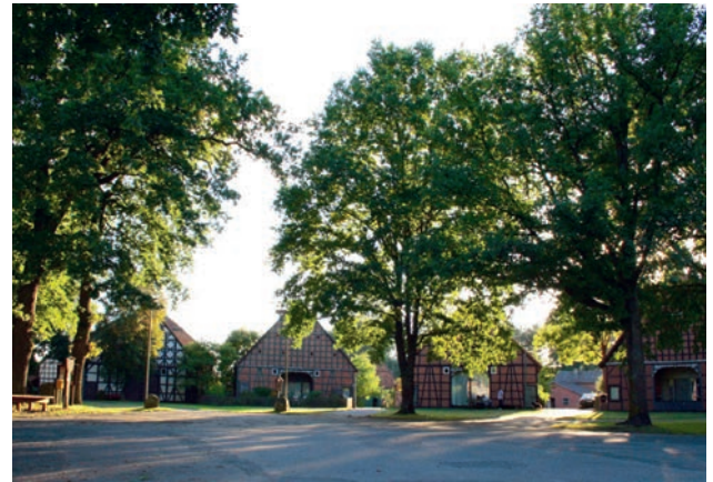
Fig. 1.11 Schreyahn, vernacular timber-framed architecture; the predominance of hall houses conveys a homogenous picture of the village (photo by Kerstin Duncker)
