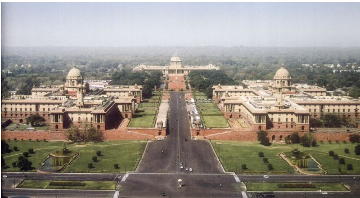
Fig. 5: New Delhi, aerial view towards west end of central axis, former Viceroy's House atop Raisina Hill flanked by South (left) and North (right) Secretariat blocks, showing dominant use of neo-classical revival style
