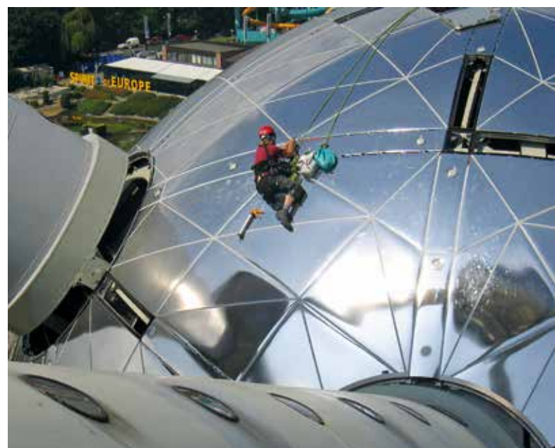
Fig. 6: Installing the meridian plates (photo Origin 2005)
