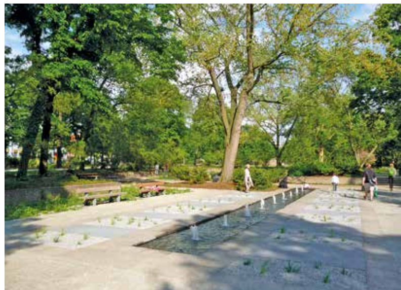
Fig. 9: Fountain basin in Kleiner Tiergarten after renovation (photo Bernd Krüger, 2016)
