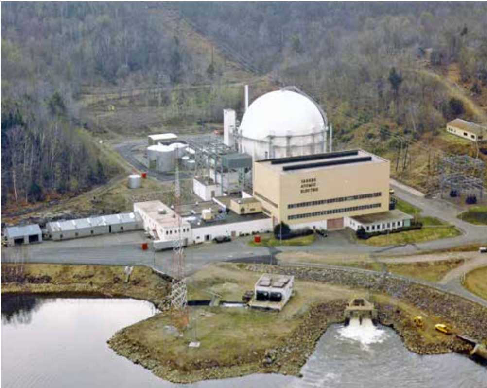
Abb. 9: Yankee Rowe Nuclear Power Station, Franklin County, Massachusetts, USA, 1957–1960.
