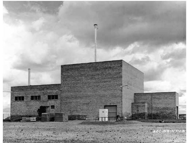
Abb. 4: Gebäude des Experimental Breeder Reactor, National Reactor Testing Station, Idaho Falls, Idaho, USA, 1950–1951.
