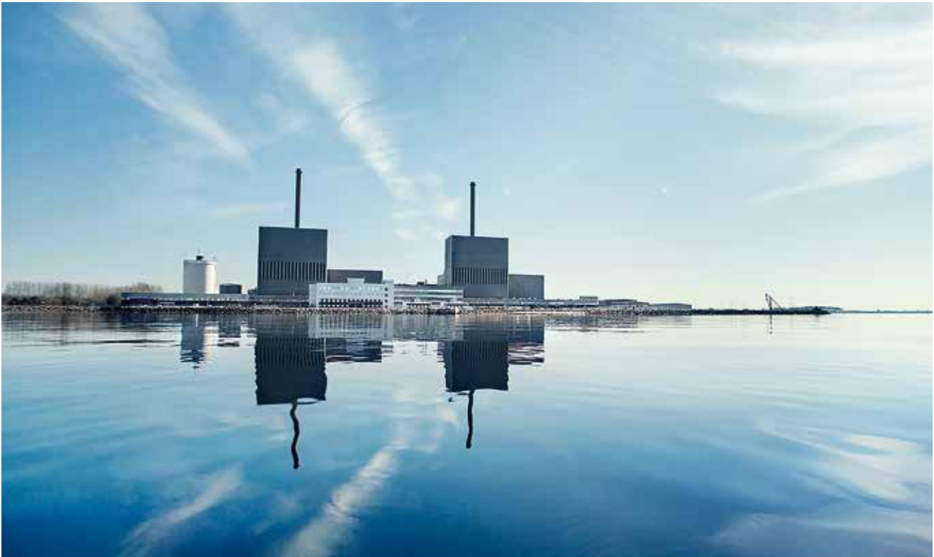
Fig. 10: Oskarshamn 1 (O1), the first light water reactor in Sweden in grand scale opened in 1972 as a private project run by OKG Group. The capacity of O1 was 400 MW. The reactor was followed by two late reactors. O1 was closed down in 2017.
