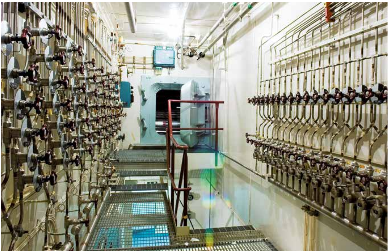
Fig. 9: Solenoid valves in the Fuel Element Failure Detection System, detail. This bank of valves is used to sequentially connect cooling water samples from the fuel elements to the fission gas scrubbers. Swedish art of engineers in the 1960s.
