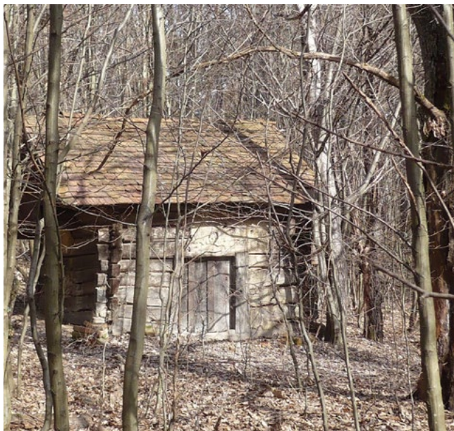
Fig. 32: Forest house near Bajánsenye built 1833
